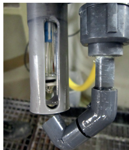
Via the nozzle, the pH+ORP sensor is flushed periodically
