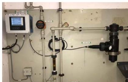
Measuring station with Liquiline CM442 transmitter and Turbimax CUS52D turbidity sensor
