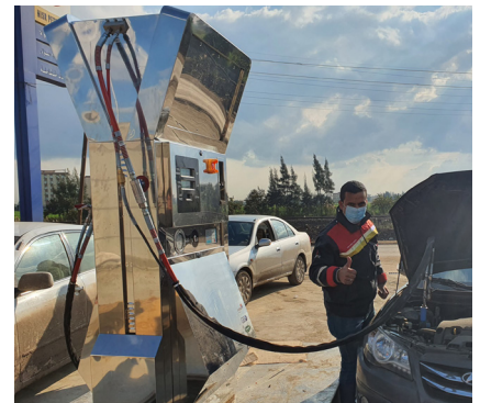
Dispenser model : Dual hose, CNG Dispenser delivered in Egypt
