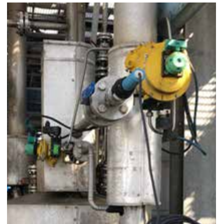
Oxygen measuring point with Memosens COS81D
