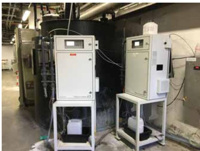
Both CA72TOC analyzers in use in outlet of biological wastewater treatment process.
