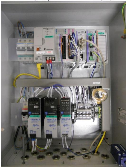
The controller consists of the following modules, mounted in a steel enclosure:
